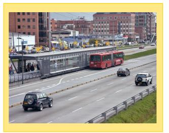
TransMilenio is a flexible bus system that uses exclusive busways to feed people into and out of the central business district (CBD). The stations are located in the middle of the road to facilitate the transfer between buses in both directions. The bus stops are 57 stations, located every 700 meters
